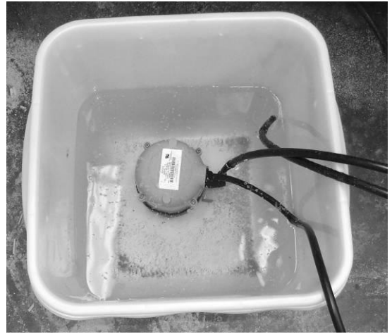
Pump in water container
