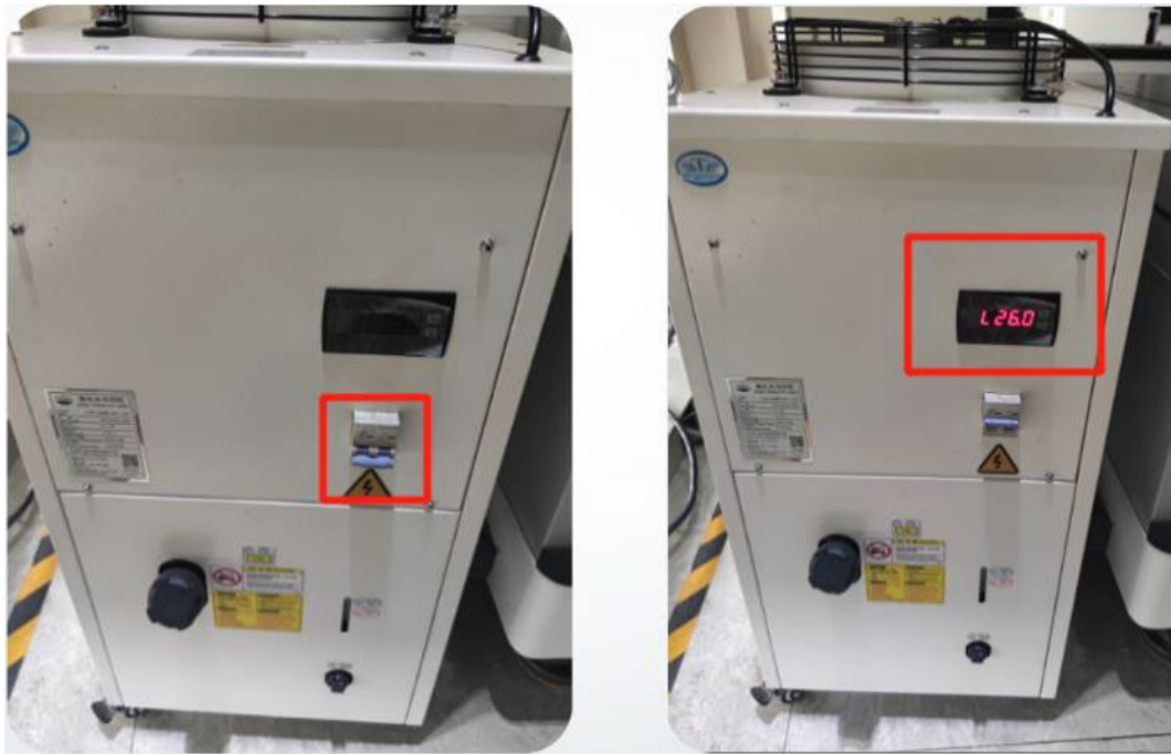
Figure 3-4: Chiller Switch
