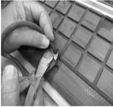
Cutting end of foam rubber gasket
