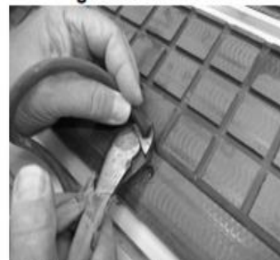
Cutting end of foam rubber gasket
