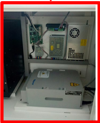
Open Back Panel of the Control System.
