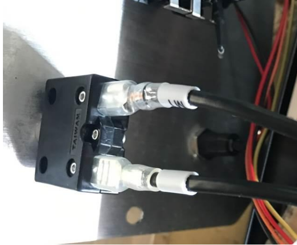
Figure 2I : Replacing circuit protector
