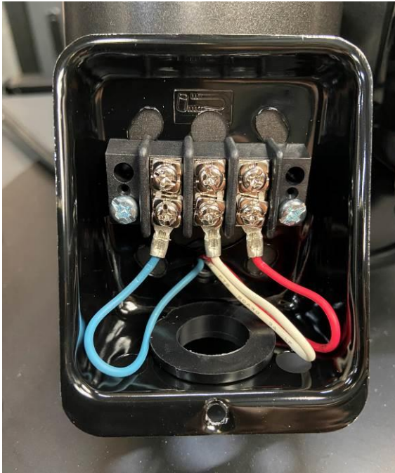
Figure 2W: 220V bottom wiring in auto clean junction box
