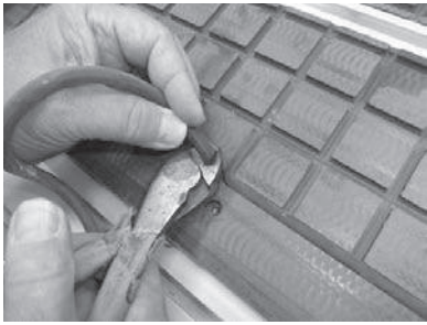
Cutting end of foam rubber gasket
