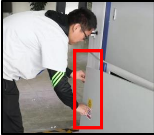
9d.) Turn on the air switch of the electrical cabinet main circuit.
